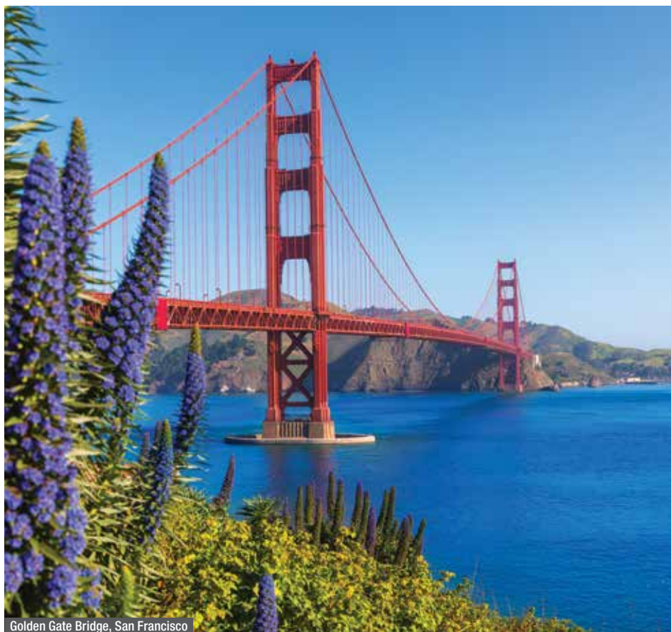
Golden Gate Bridge, San Francisco
